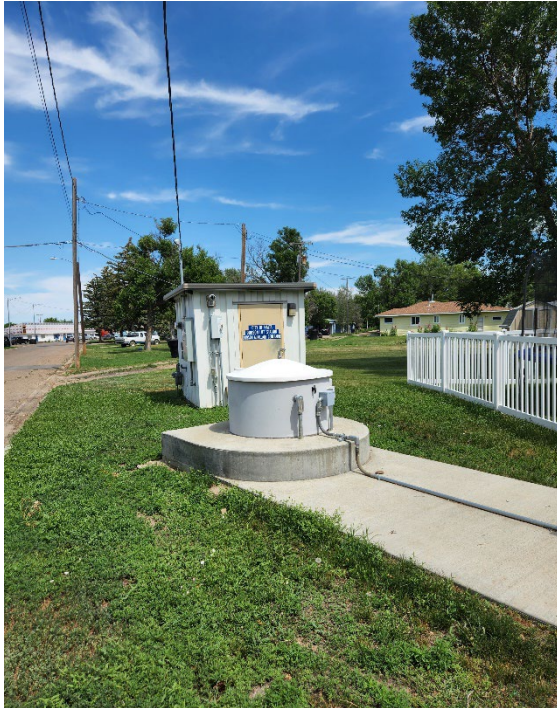
Figure 3 - Dobson Lift Station
