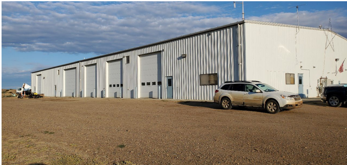
Figure 11 – City Shop Building
