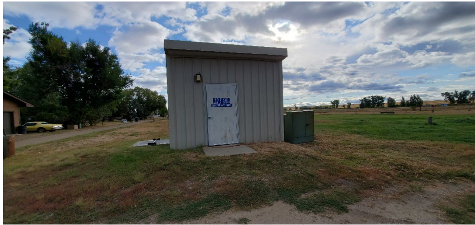
Figure 13 - Legg Storm Pump Building
