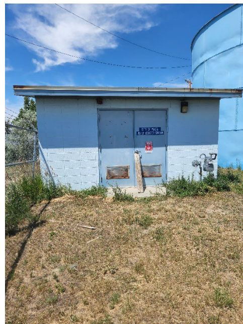
Figure 9 - Water Booster Station
