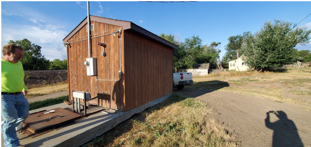
Figure 2 - West Side Lift Station
