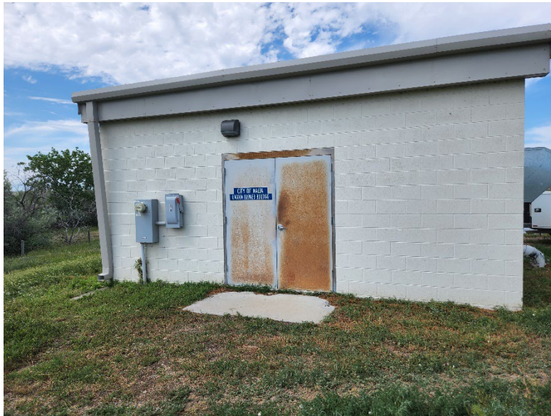
Figure 5 - Blower Building at Lagoons
