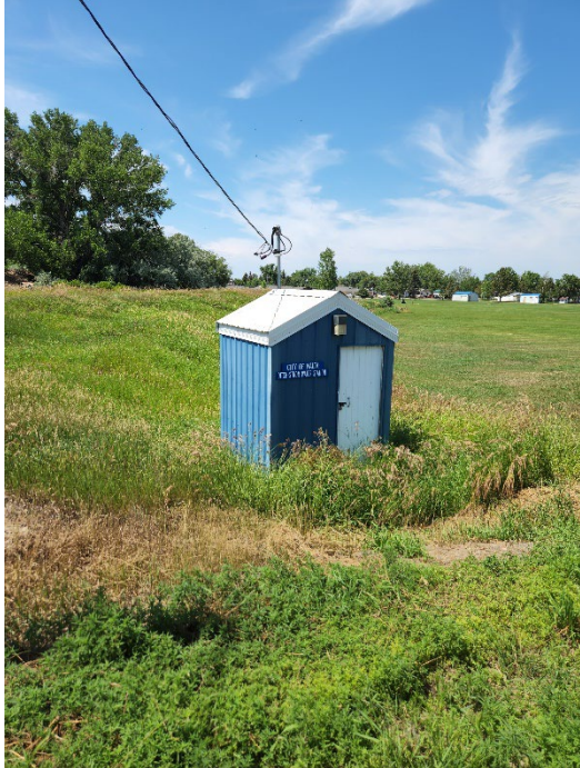
Figure 15 - Ditch Storm Drain Pump Station
